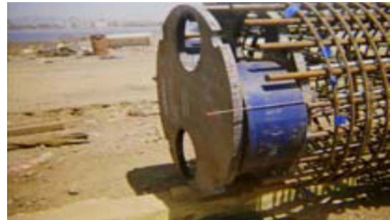
Fig. 5 Test Pile 2113-1 lower O-cell assembly
