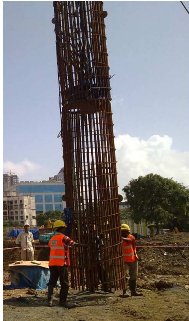
Fig. 12 O-cell assembly welded to Test Pile 2873-1
