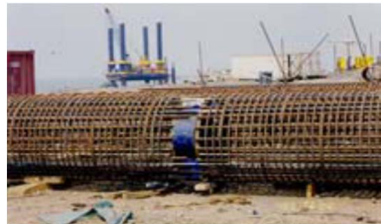
Fig. 6 Test Pile 2113-1 upper O-cell assembly
