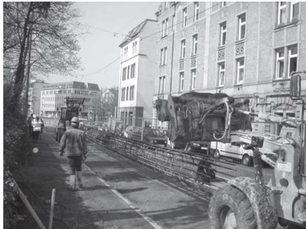
**Fig. 8** Carrying the pile cage to the bore on the pathway
