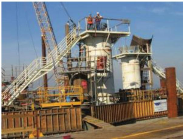
(a) Casing projections enable maintenance of head on slurry
