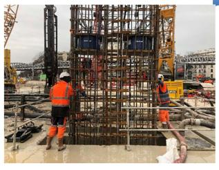
Fig. 4. Insertion of the reinforcement containing the O-cell assembly.
